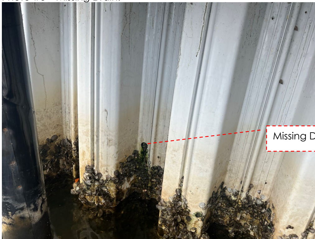
Photo #5 – Missing Drain.
