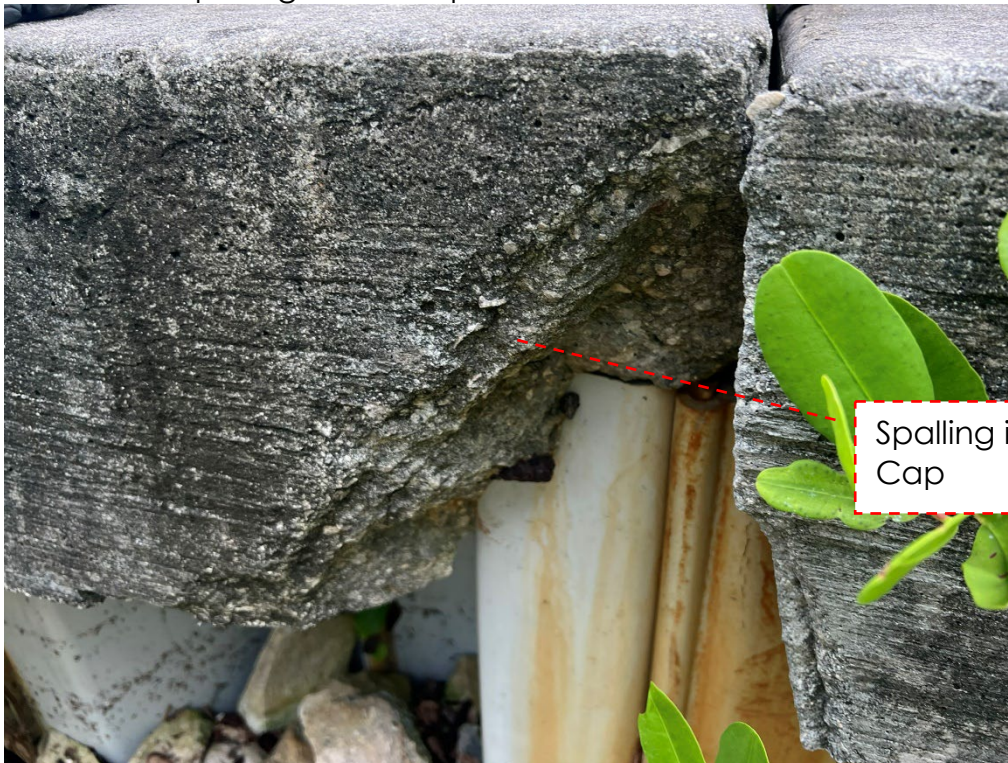
Photo #4 – Spalling in the Cap.
